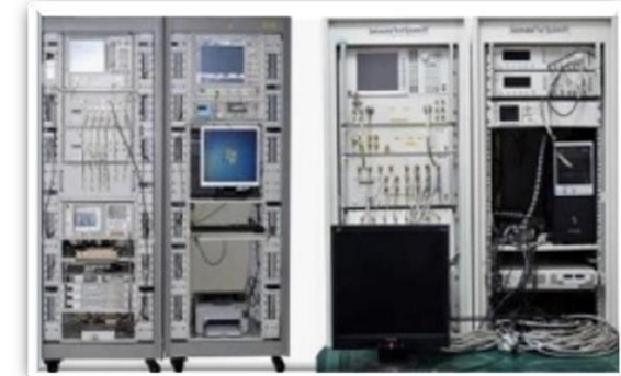
ATE ATS - Facility
