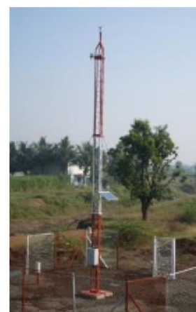
Weather Monitoring Station
