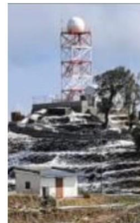
Meteorology Radar Systems
