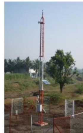
Weather Monitoring Station
