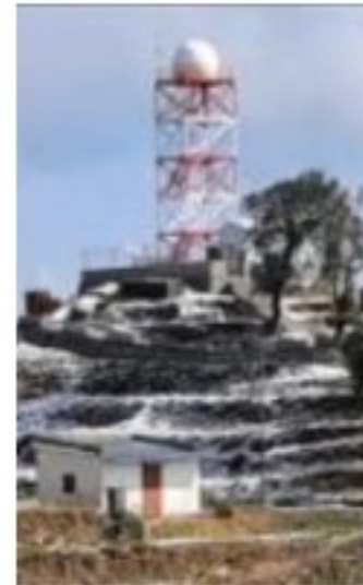
Meteorology Radar Systems
